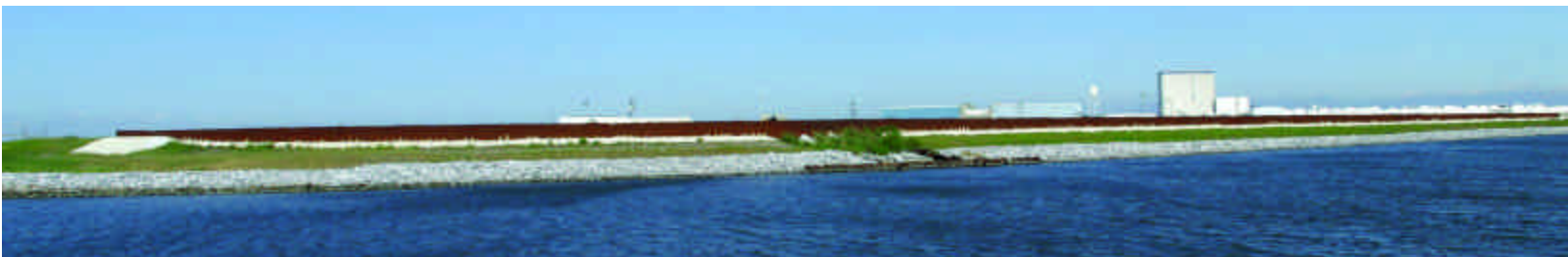
View from the East of Michoud's levee protection
