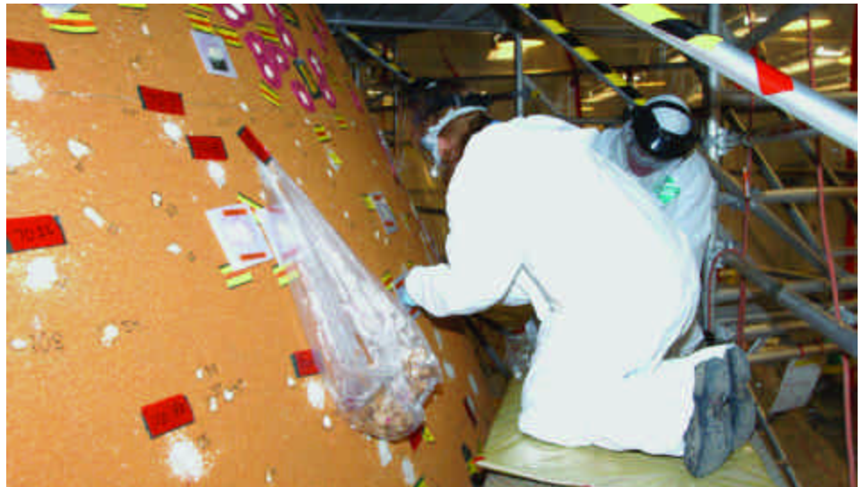
In KSC's Vehicle Assembly Building, USA technicians Brenda Morris (left) and Brian Williams apply foam and molds to areas damaged by hail on ET-124. The red material is sealant tape so the mold doesn't leak when the foam rises against the mold.
